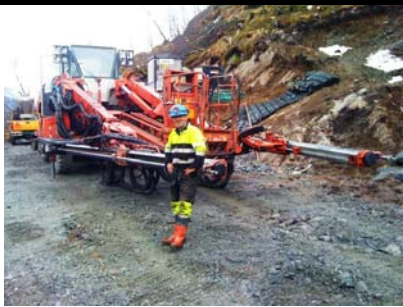
Tamrock Tunnel drilling rig
