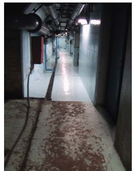
Turbine corridor in painting process
