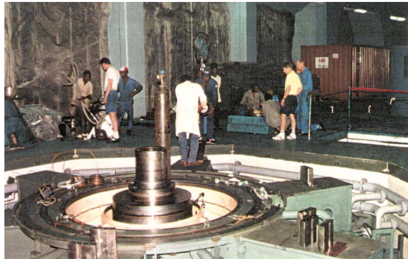
Generator under rehabilitation
