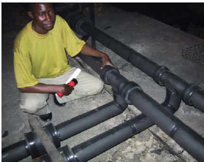
New pipeline insulation
