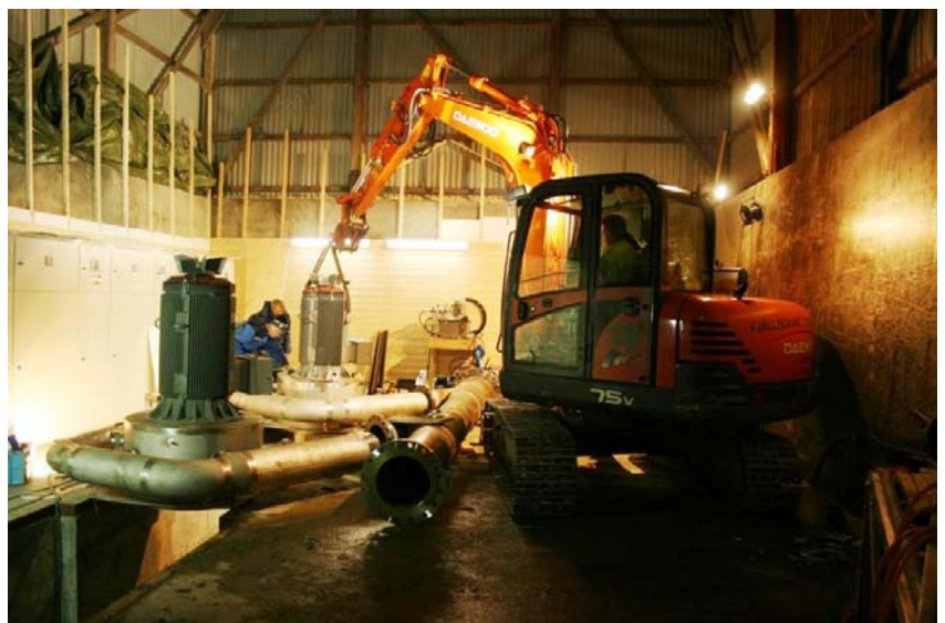
Turbines and generators during assembly
