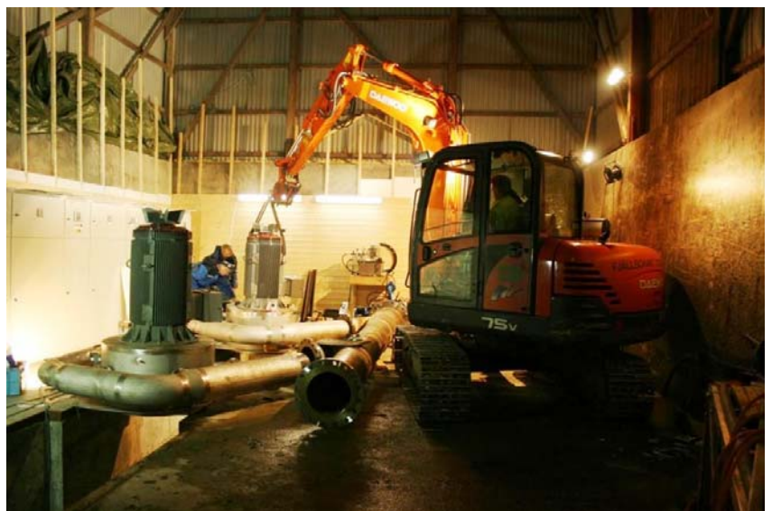
Turbines and generators during assembly
