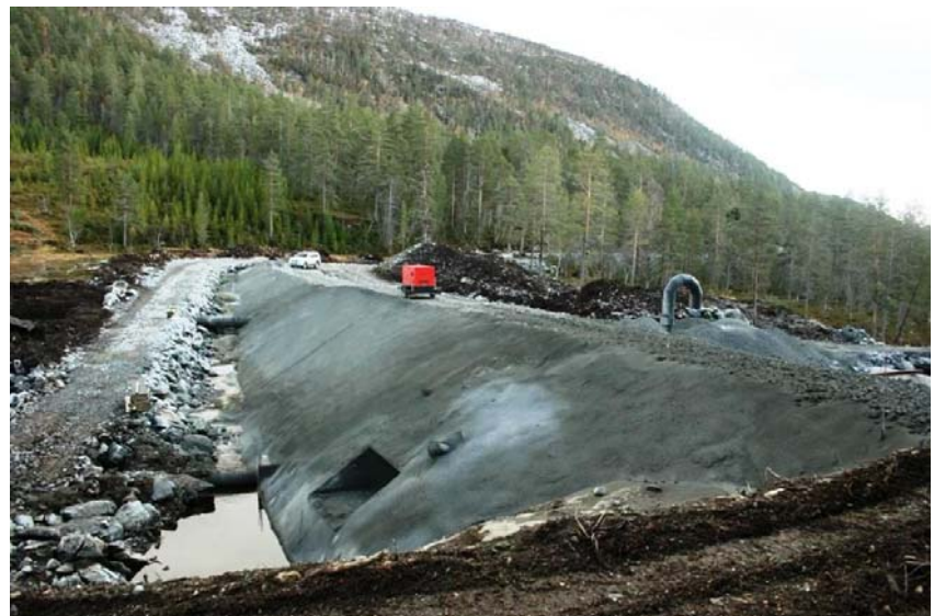
Dam and intake structure
