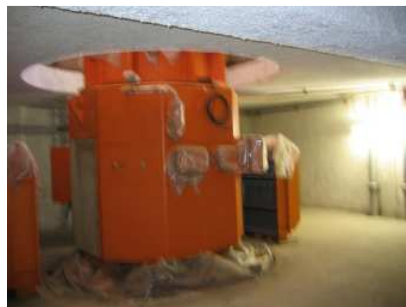
Only generator & turbine erected
