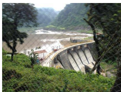
Santa Maria intake just below
